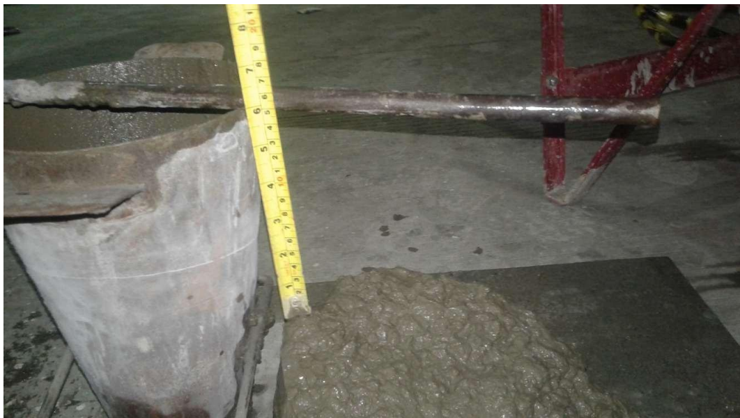
Gambar 6. Uji Slump Beton ( Slump Test )
