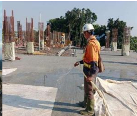
Gambar 9. Curing Beton Lantai
