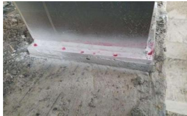
Gambar 36. Non-Destructive Test (Baja)
