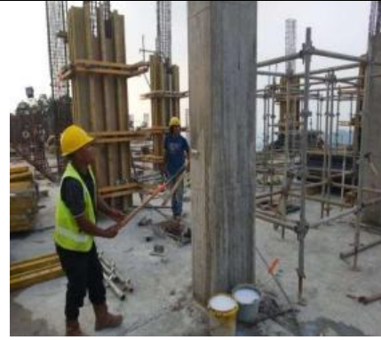
Gambar 15. Curing Compound Beton Kolom
