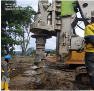
Gambar 4. Pengeboran Bored Pile
