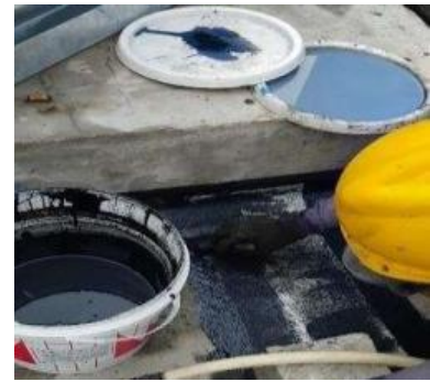
Gambar 33. Pek. Waterproofing
